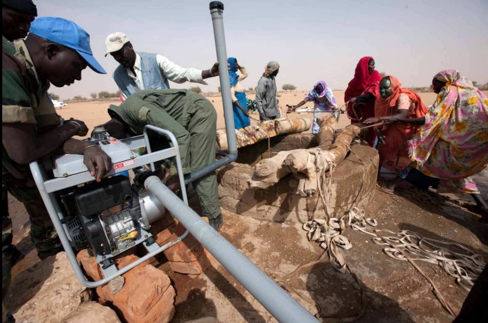
Construction of Water Pump for Well -- North Darfur, Sudan
